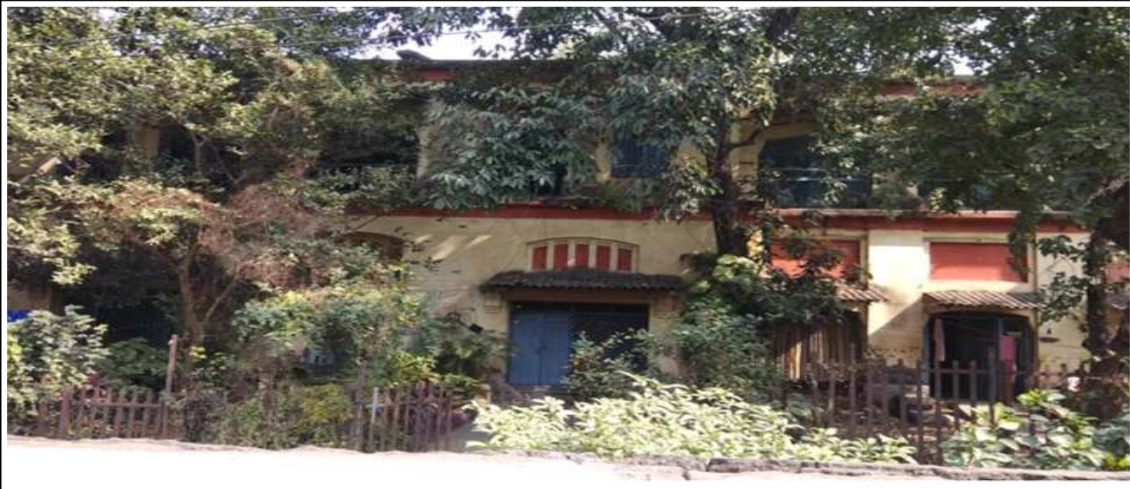
Heritage Structure of Old DS's Bungalow-cum-Office
