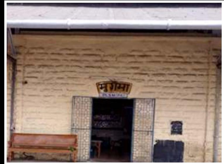
Mugma Station Building
