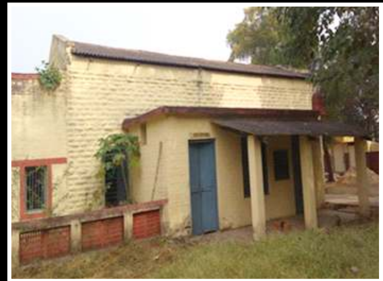
Kalubathan Station Building
