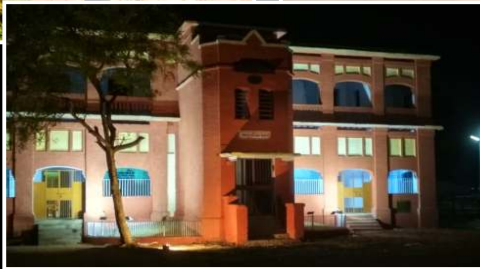
Heritage Structure of Old European Institute, Madhupur before & after renovation
