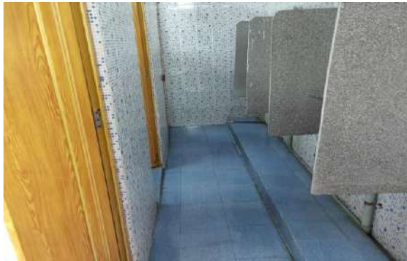
Cleaned urinals at Mysuru station
