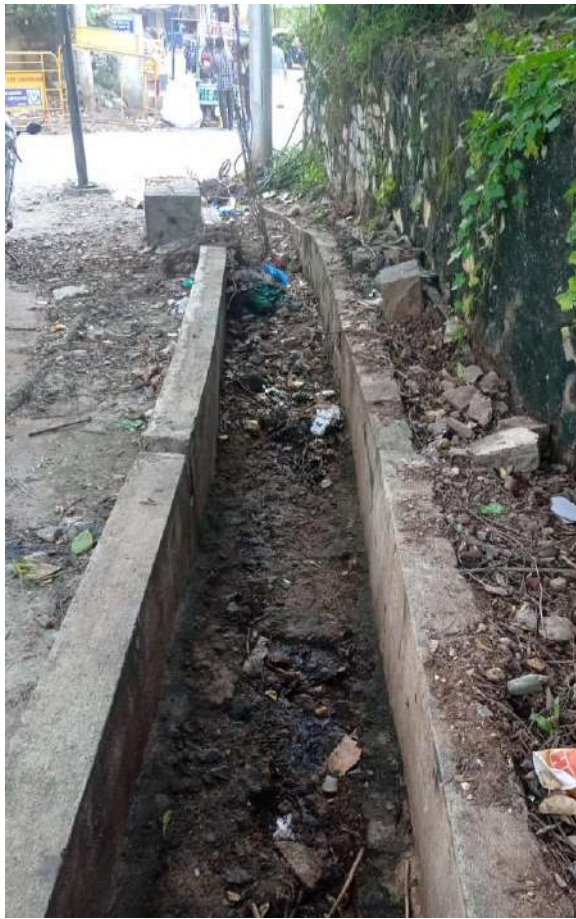
Before cleaning at Davangere station
