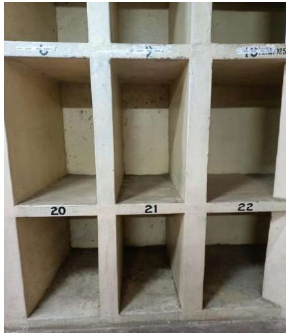
After cleaning Sr.DMM office Mysuru
