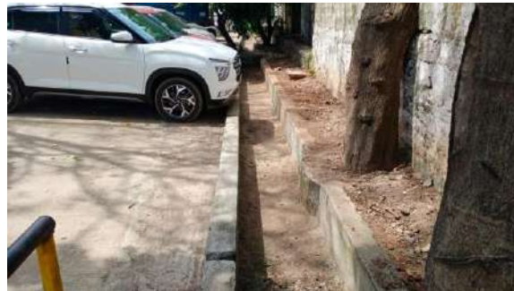
Cleaned drainage at Davangere station
