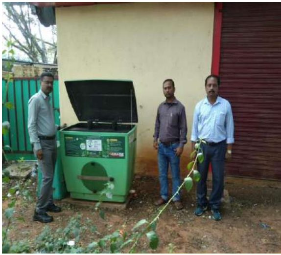
Inspection of Composter at Arasikere station
