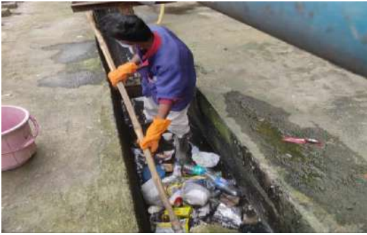
Intensive cleaning of drainage at Mysuru station
