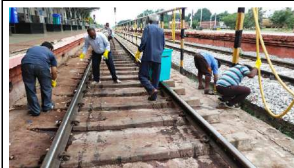
Intensive track cleaning at Harihar station
