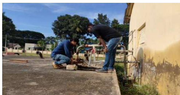
Inspection of GLR at Arasikere station
