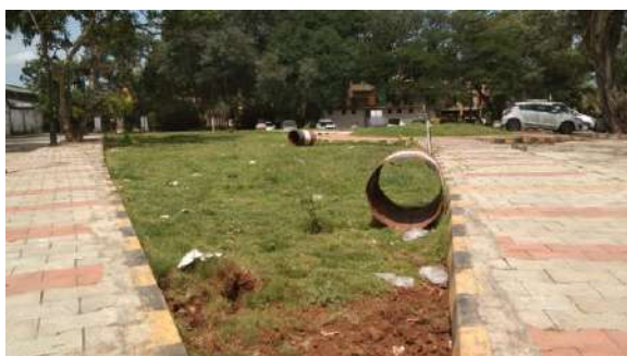
Before cleaning at Davengere station
