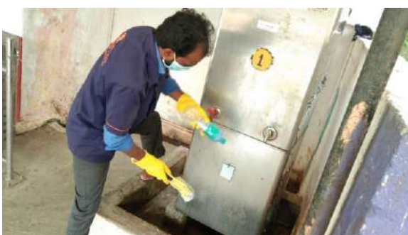
Intensive cleaning of water coolers at Davengere station
