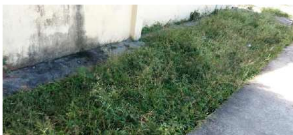
Before cleaning at Shimoga colony
