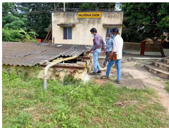
Inspection of water tanks at Mysuru colony by CHI Division
