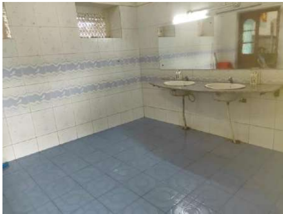
Cleaned waiting room wash area at Mysuru station
