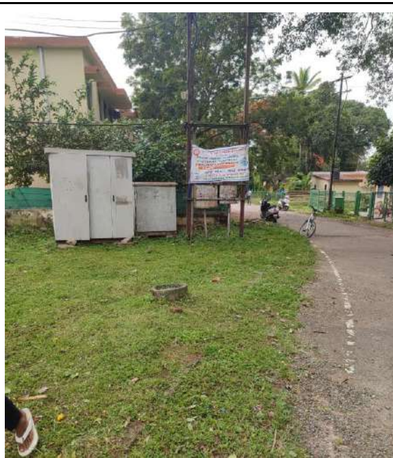
After cleaning at Mysuru colony
