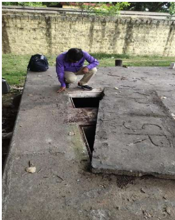
Inspection of water tank at Harihar station by ACMS
