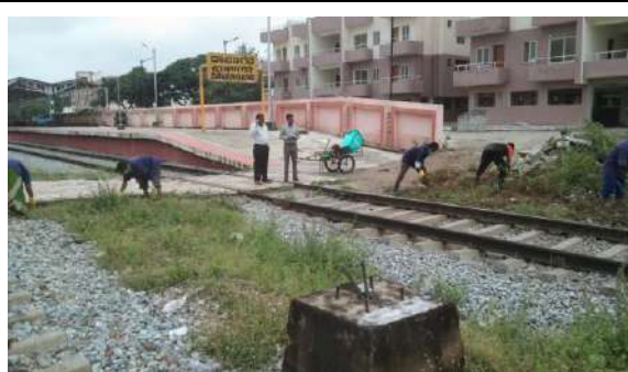
Inspection of tracks at Davengere station by ADSTE and CHI
