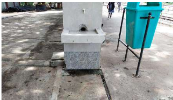
After cleaning at Harihar station
