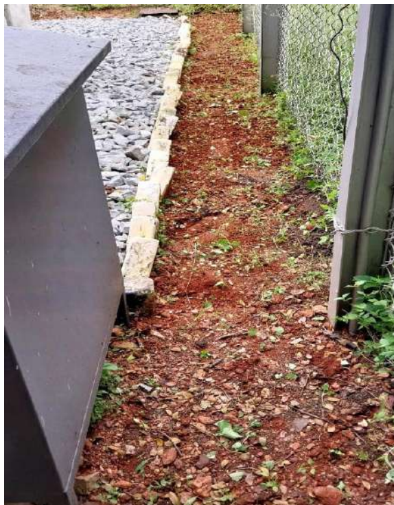
After cleaning inside Birur sub station
