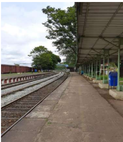
Cleaned tracks at Sakaleshpur station
