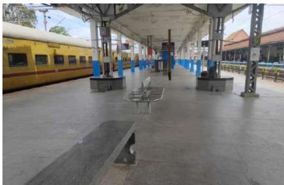
Litter free platform at Mysuru station
