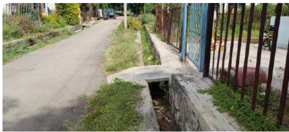
Before cleaning at Arasikere station
