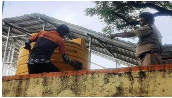
Cleaning of water tank at SMET by RPF
