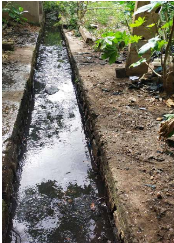
Sakaleshpur drainage after cleaning
