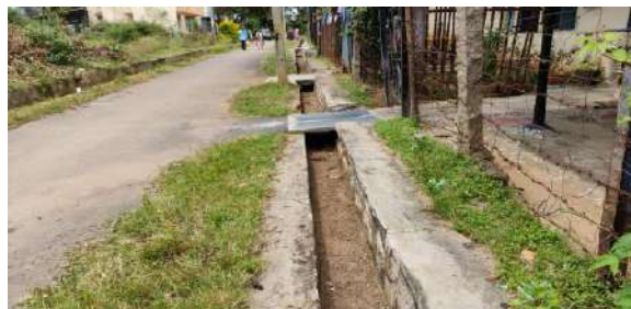
After cleaning at Arasikere station
