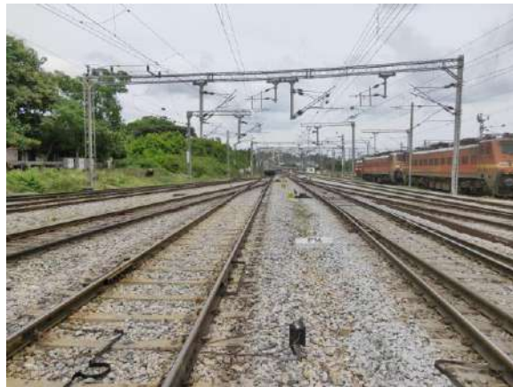
Cleaned tracks at Mysuru station
