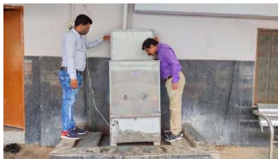
Inspection of water coolers at Harihar station by ACMS/HRR
