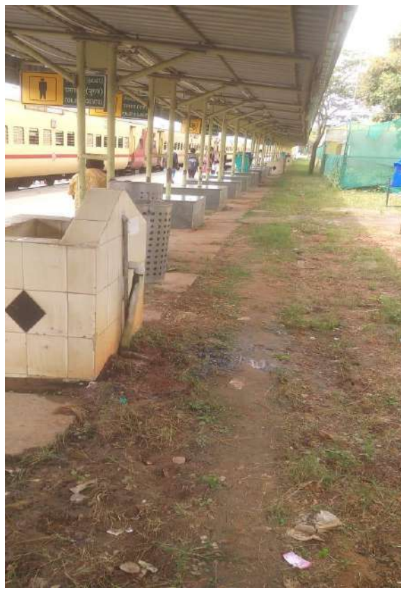
Deweeding done at Hassan station
