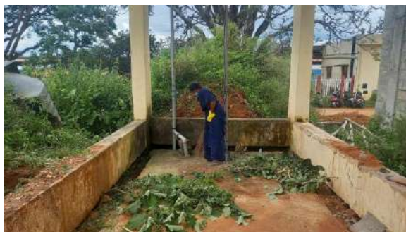
Cleaning of water tank at Ashokapuram
