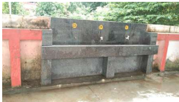
After cleaning of water taps at Davengere station
