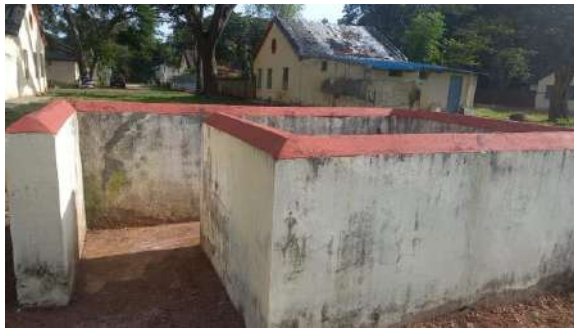
Cleaned dustbin at Ashokapuram colony
