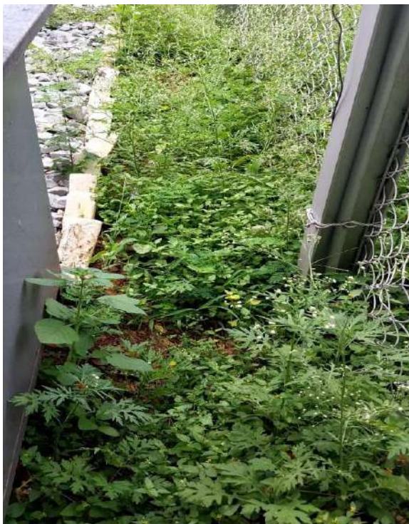
Before cleaning inside Birur sub station
