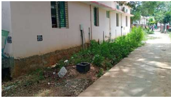
Before cleaning at Davangere colony
