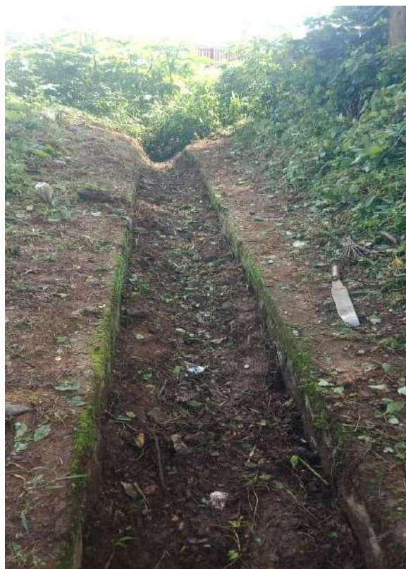
Sakaleshpur drainage after cleaning
