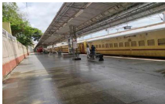
Cleaned platform at Mysuru station
