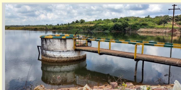
Devaragudihal Lake, one of the largest water bodies in Indian Railways with a capacity of 1935 Million Litres near Hubballi revived in 2021
