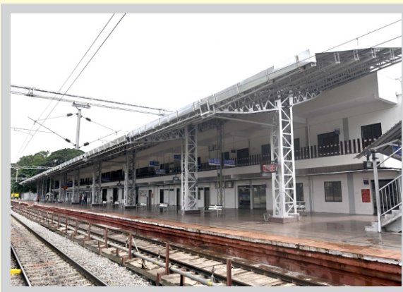
Platform Shelter at Dharwad
