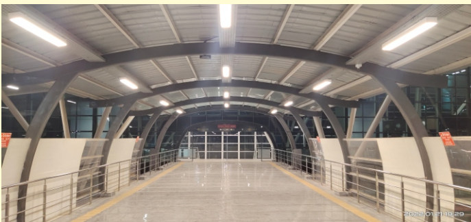
Foot Over Bridge
