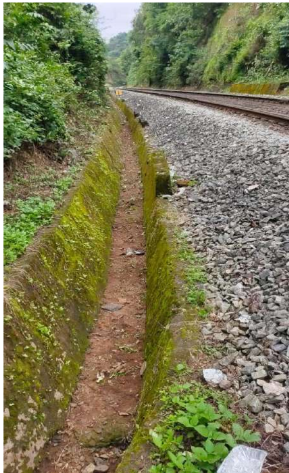
Intensive cleaning of open drains near tracks at Subramanya road section
