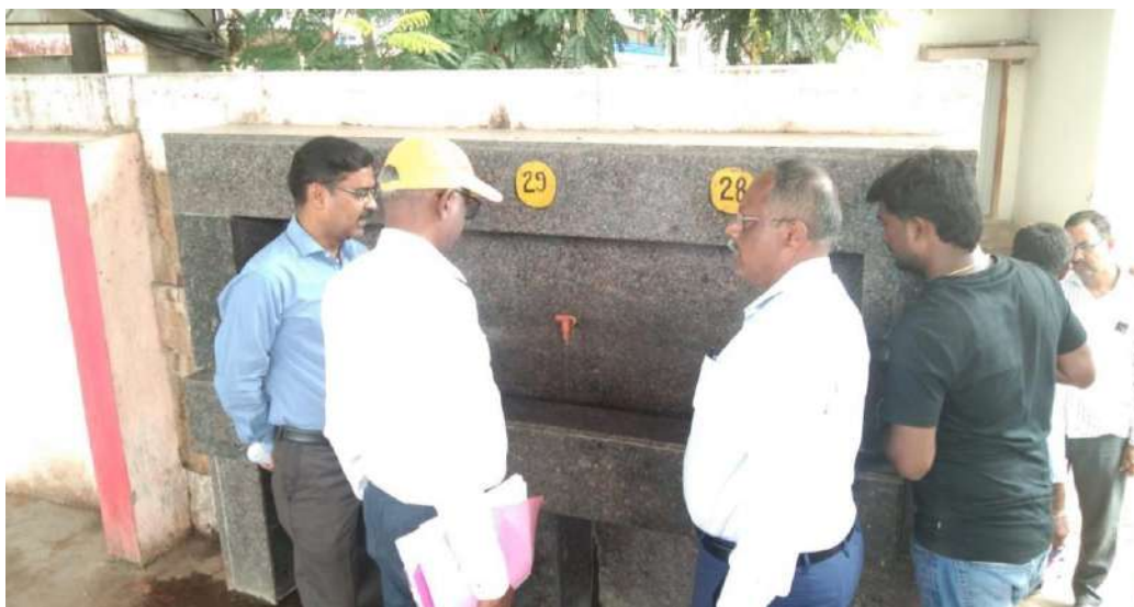
ADEN/DVG,SSE/W/DVG and CHI/DVG inspected water supply pipe lines and quality of water is checked at DAVANGERE station
