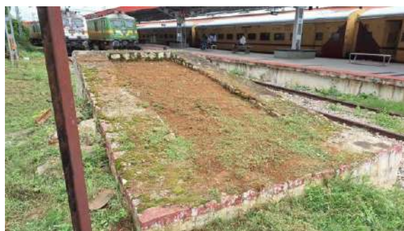
Mysuru station after cleaning
