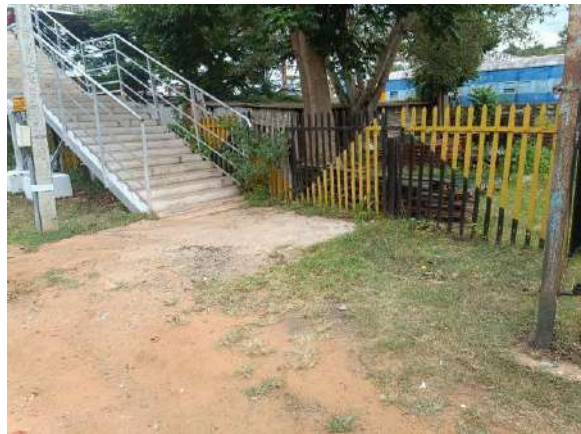
After cleaning at Arsikere station
