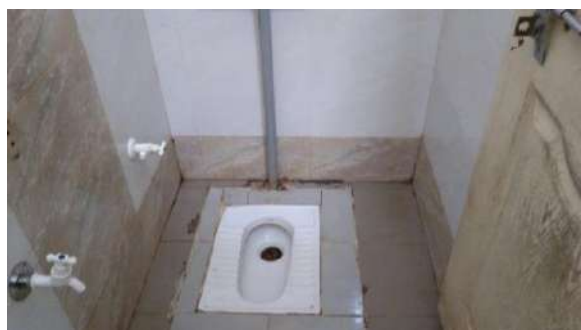
Cleaned toilet at Davangere station
