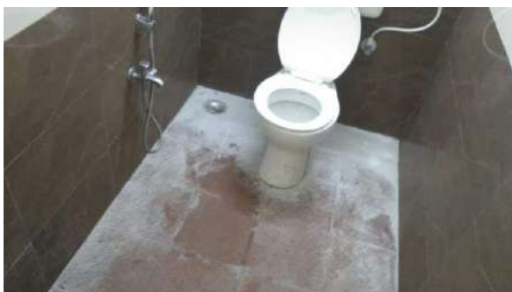
Before cleaning of Retiring room toilet at Davangere station
