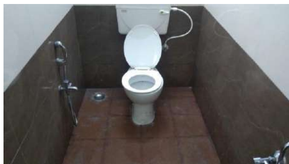
After cleaning of Retiring room toilet at Davangere station
