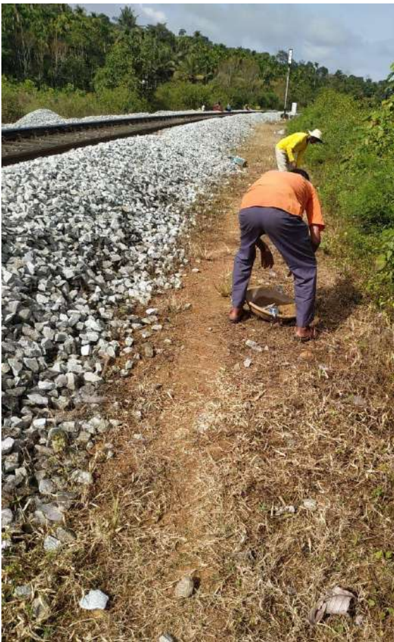
Intensive cleaning of tracks at ghat section Sakleshpur
