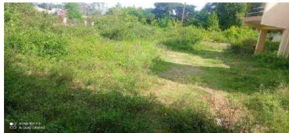
After cleaning at Mysuru Loco colony
