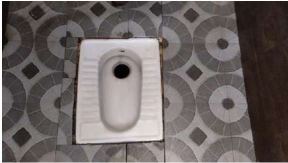
Harihar toilet after cleaning
