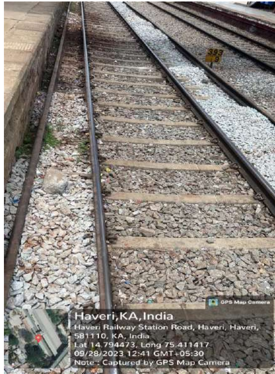
Cleaned track- Haveri station
