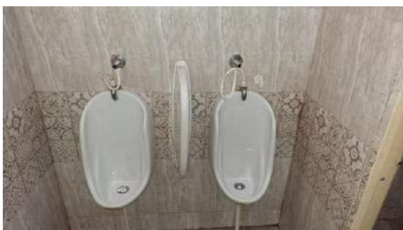
Cleaned urinals at Mysuru station
