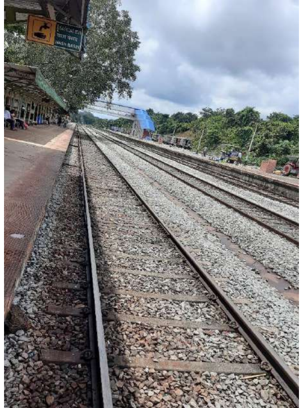
Litter free tracks at Subhramanya road station
