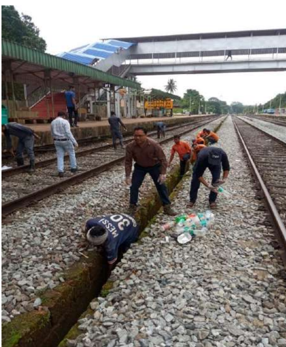
Special cleaning of tracks at Subramanya road station
