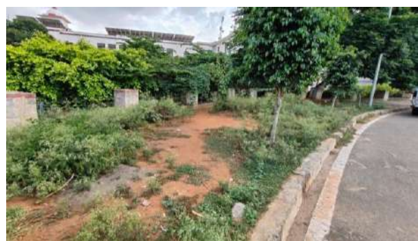
Mysuru station approach road- Before Cleaning
