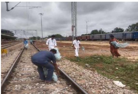
Track During cleaning at CHITRADURGA station
