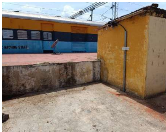
After intensive cleaning at Arsikere station
