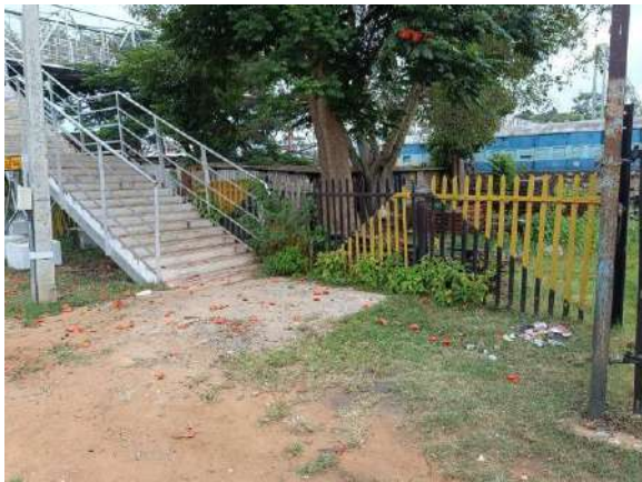
Before cleaning at Arsikere station
