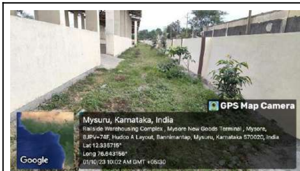
MNGT compost plant before
