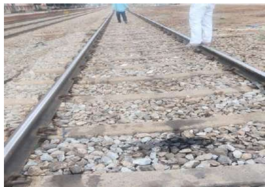
Track after cleaning at CHITRADURGA station
