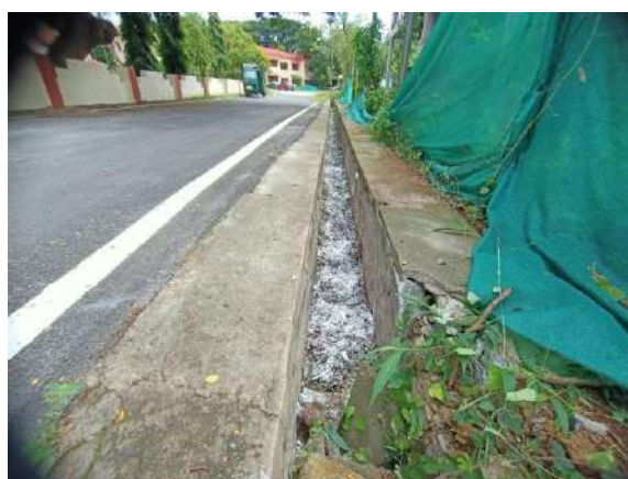
Mysuru colony open drain after cleaning
