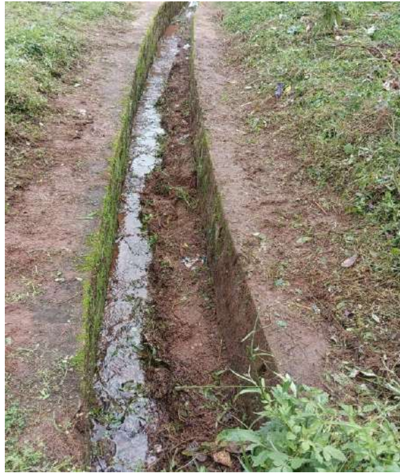
Sakaleshpur colony drain after
