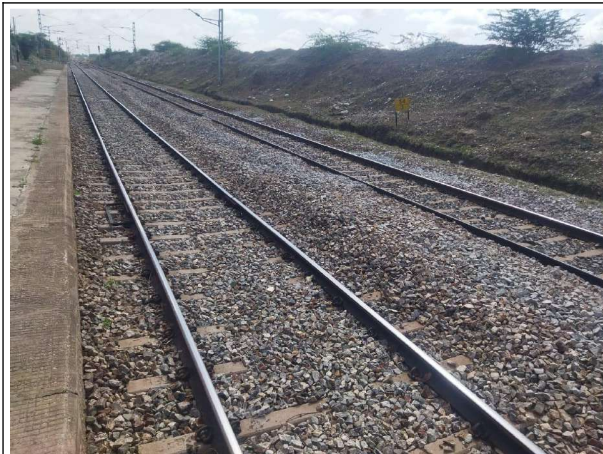
Cleaned tracks of Balenahalli station
