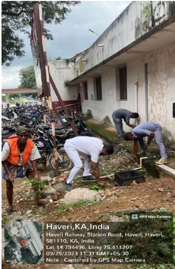
During cleaning-Haveri station
