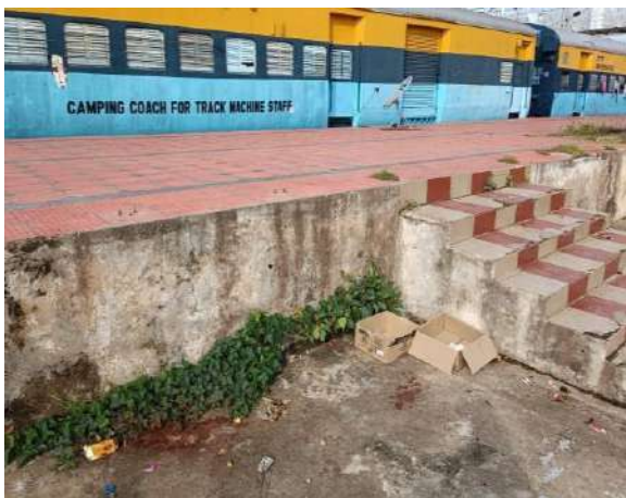
Before intensive cleaning at Arsikere station
