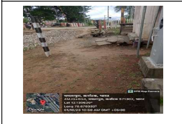
Cleaned track area at Nanjangud Town
