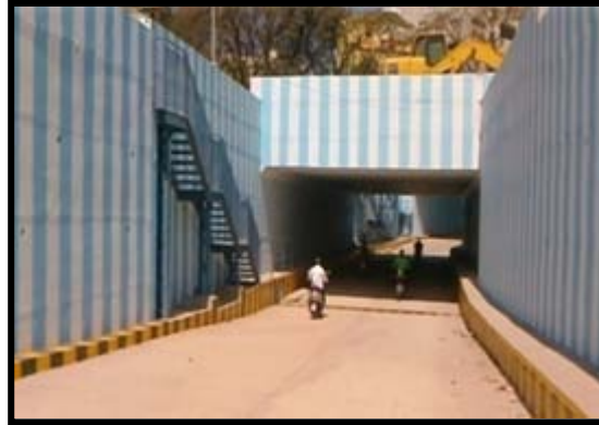
Road Under Bridge between KSR Bengaluru and Nayandahalli
