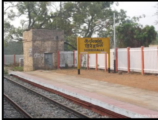
Raising and Extension of Rail Level Platforms Hirehalli Station
